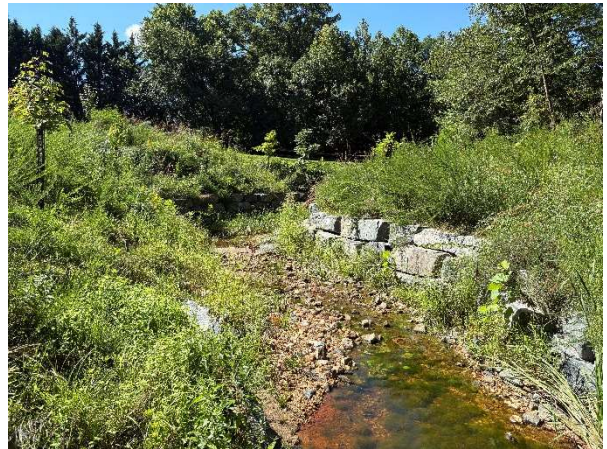
Photo Station 10 (2025): From last structure looking downstream. Imbricated boulder wall on either side of the channel. A cobble lined drainage channel is entering from the right bank (labelled as a wetland on plans). Low flow in stream with high algae and iron flocculant growth. Finer deposition near culvert.
