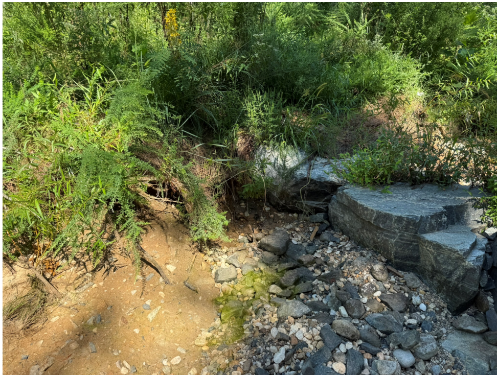
Figure 6: Erosion by step pool structures
