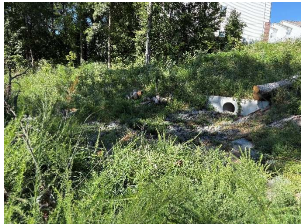
Photo Station 08 (2025): From left bank looking at stabilized banks and repaired right bank stormwater outfall. Instream bars now vegetated and common across stream. Large tree fall at outfall, but has been cut. Debris remains in pile on both banks.
