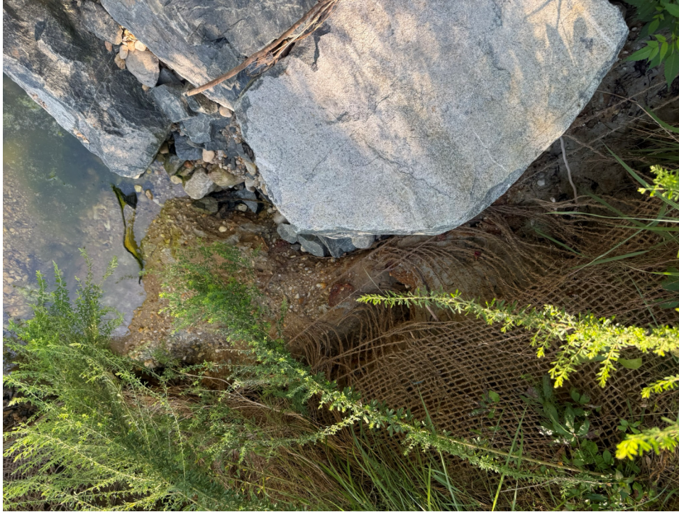
Figure 5: End around erosion around step boulder
