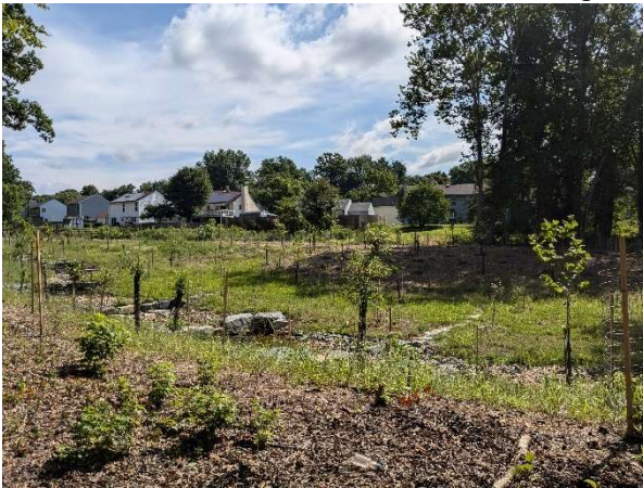
Photo Station 07 (2024): From right bank looking at channel. Wide floodplain bench on the left bank. Vegetative establishing but some bare patches near tree plantings; near forested wetland on right bank. Drainage channel on the left hillslope is causing some erosion.
