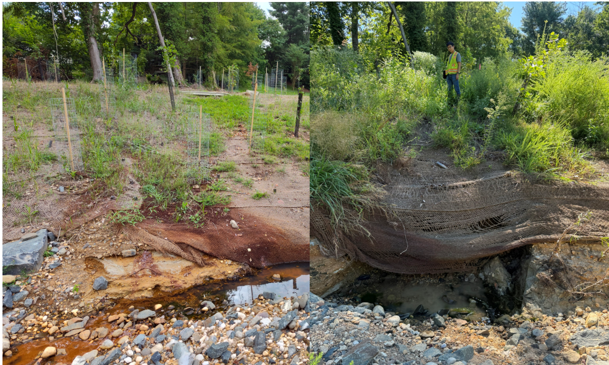
Figure 2: Severe bank erosion from hillside seep. 2024 conditions on left, 2025 conditions on right. Biohabitats team member standing near uphill extent of erosion.
