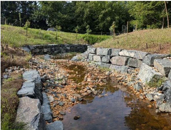
Photo Station 10 (2024): At last structure looking downstream. Imbricated boulder wall on either side of the channel. A cobble lined drainage channel is entering from the right bank (labelled as a wetland on plans).
