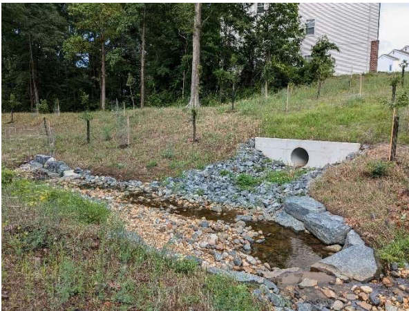
Photo Station 08 (2024): From left bank looking at stabilized banks and repaired right bank stormwater outfall. Gravel sediment bar in middle of channel is common across the stream.
