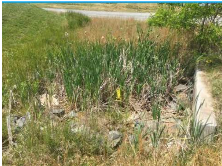
Figure B-5.8-2: Outfall Riprap and Weeds, etc.
