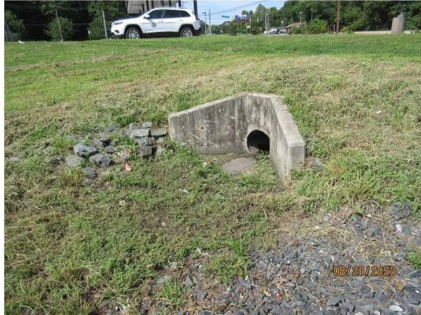
Figure B-2.4-1: Inlet Headwall
