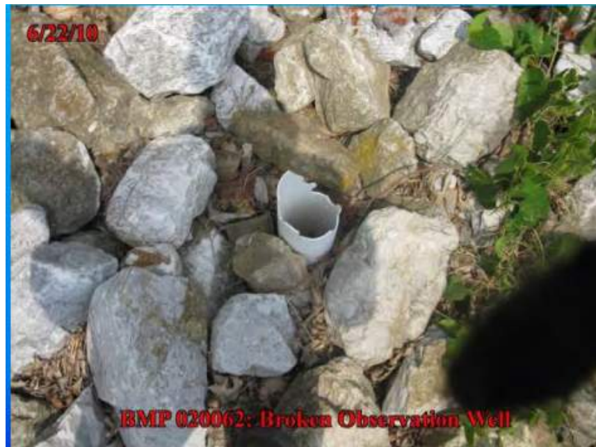
Figure B-6.1-2: Observation Well – Top Damaged
