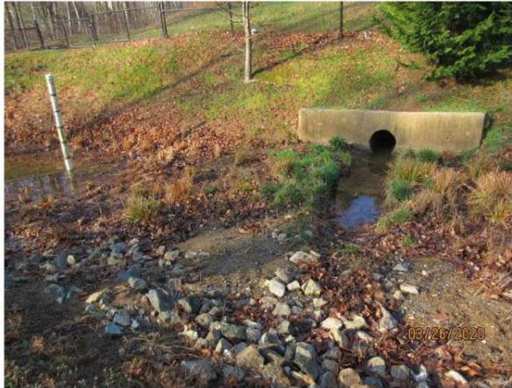
Figure B-3.3.1-1: Sediment Accumulation in Forebay (Sediment Marker Present)
