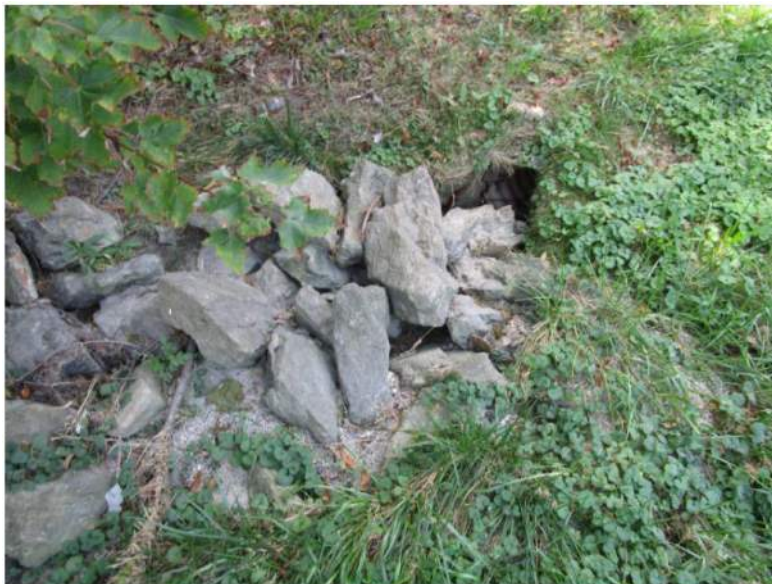
Figure B-2.4-2: Inlet Pipe Blockage
