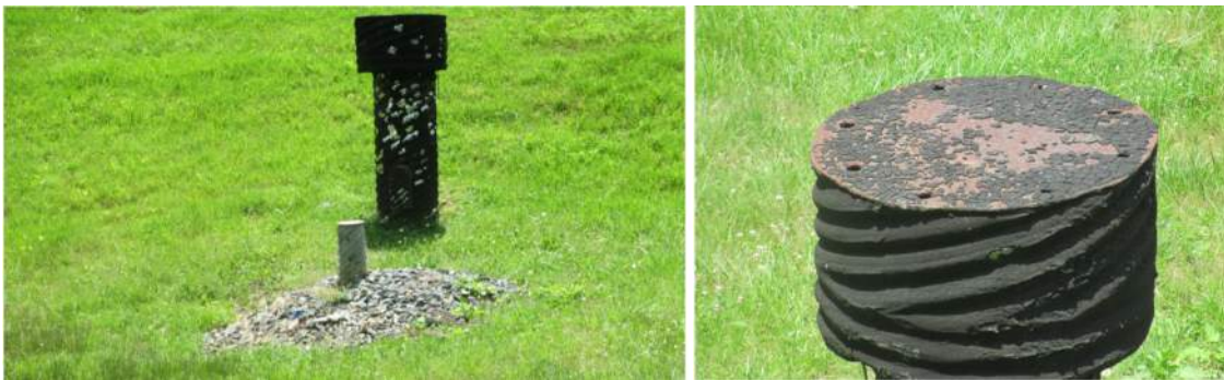
Figure B-5.1-2: Riser-Control Structure
