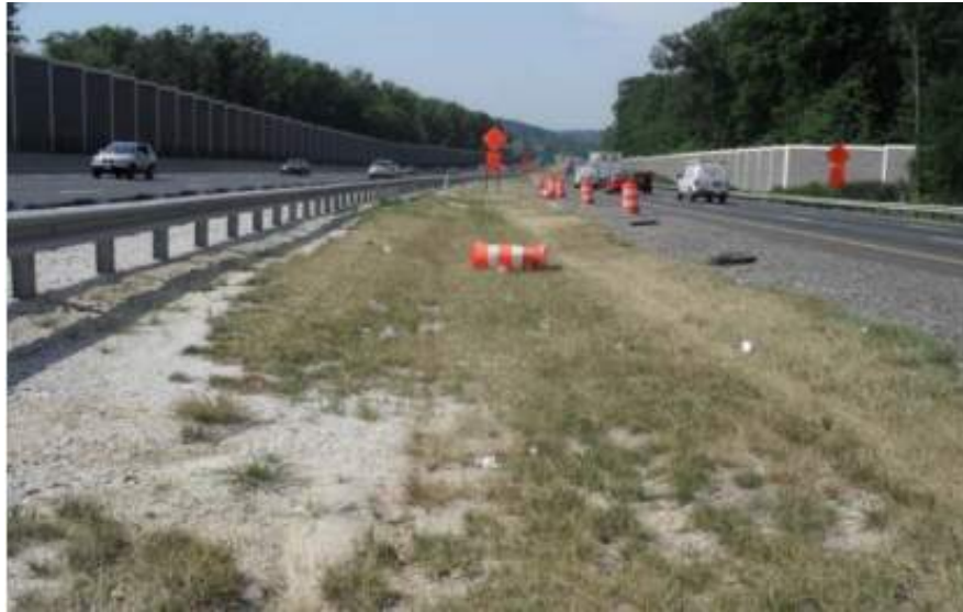
Figure B-4.5-2: Small Area of Bare Soil in Grass Swale
