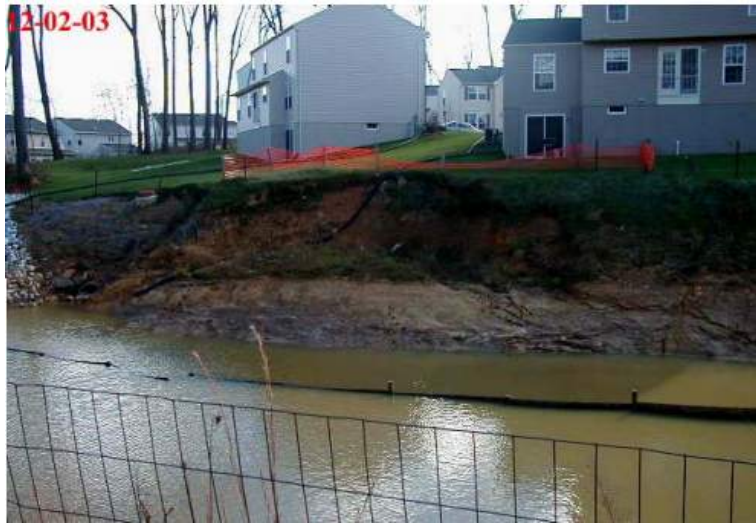
Figure B-1.1-1: Significant Failure Pond Embankment
