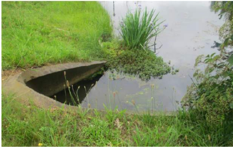
Figure B-3.1.2-1: Forebay Flooded
