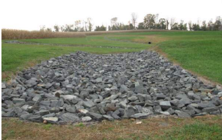
Figure B-5.9-1: Emergency Spillway
