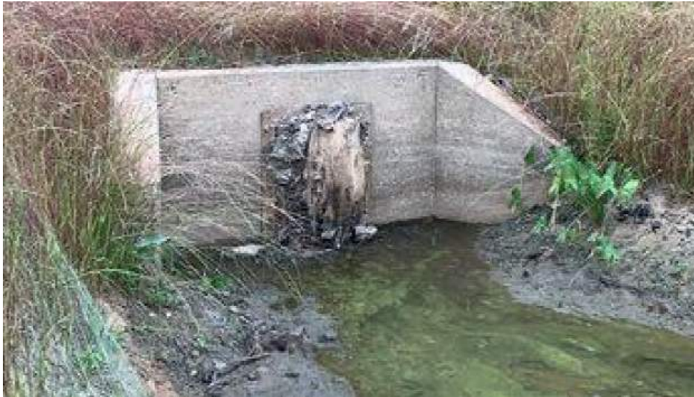
Figure B-5.3-3: Trash Racks Blocked with Debris Source: Harford County Stormwater Management Inspection Reports
