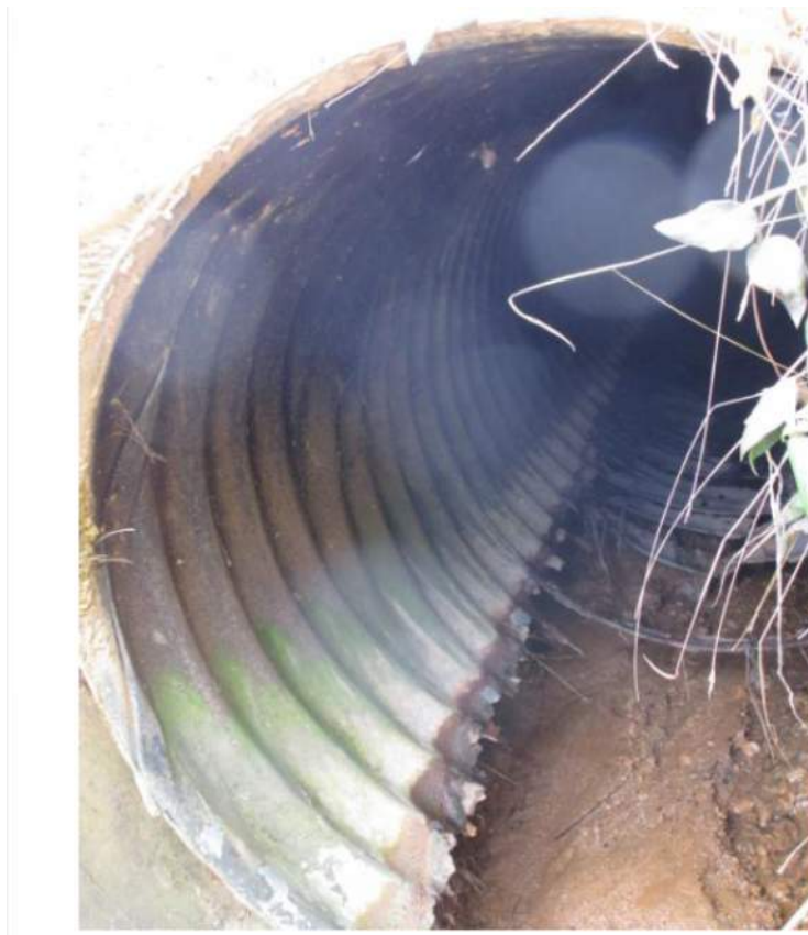
Figure B-1.3-2: Significant Failure Outfall Pipe
