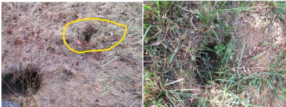
Figure B-4.2-3: Embankment Animal Burrows
