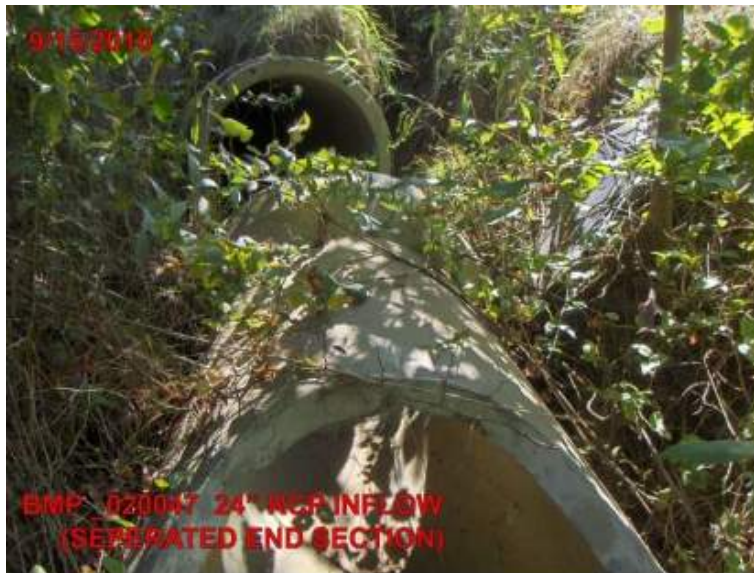
Figure B-2.3-3: Inflow Pipe End Structure Separated
