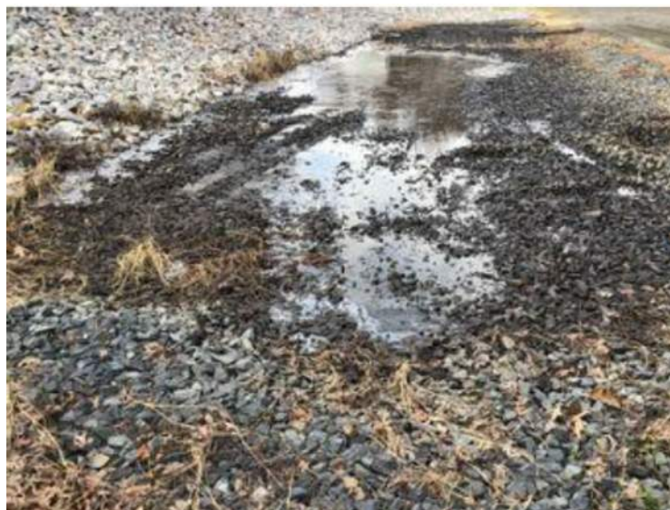
Figure B-4.1-2: Surface Standing Water
