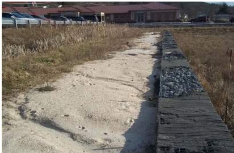
Figure B-3.3.1-2: Major Sediment Accumulation in Forebay
