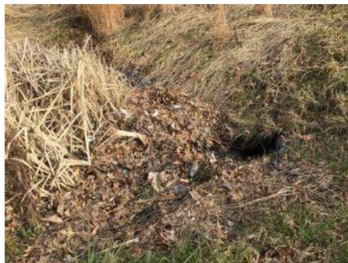
Figure B-2.1-1: Inflow Debris/Blockage Source: Harford County Stormwater Management Inspection Reports
