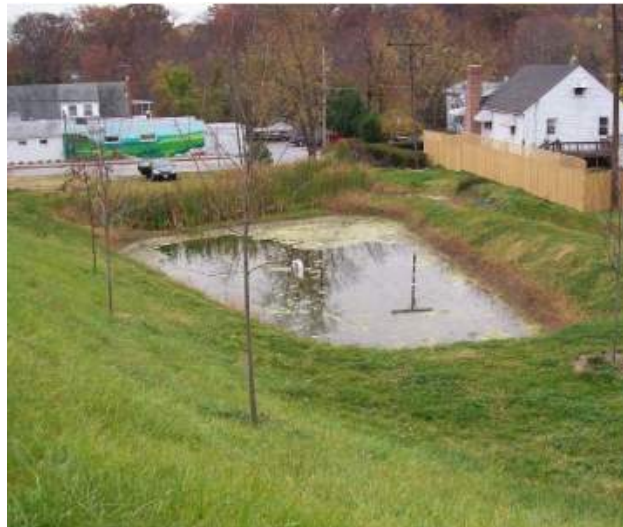
Figure B-4.1-3: Surface Sand Filter Ponding – Not Draining
