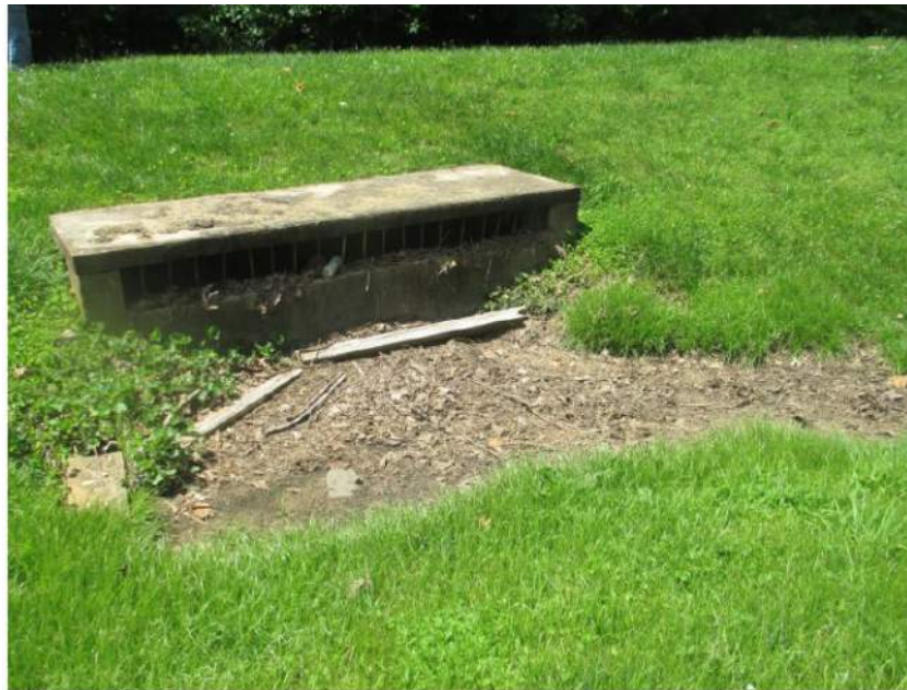
Figure B-5.1-1: Riser-Control Structure
