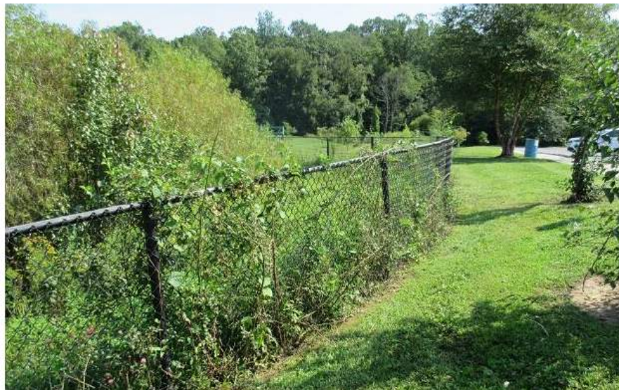
Figure B-4. 7-2: Remove Vegetation from Fence
