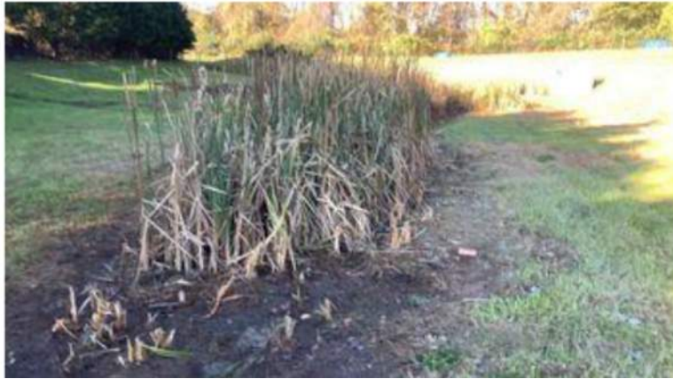
Figure B-2.2-1: Inflow Sedimentation
