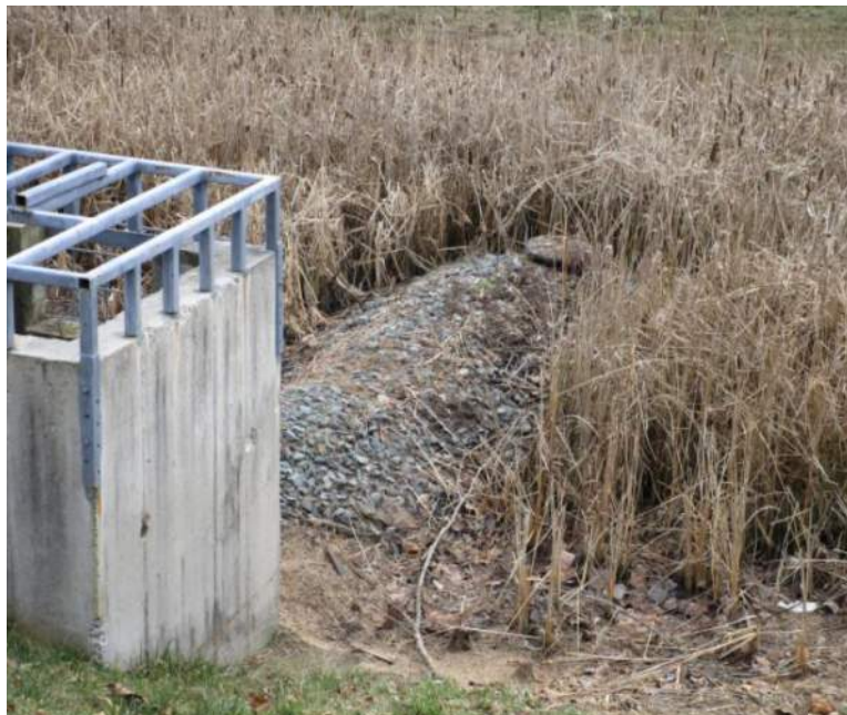
Figure B-5.5-1: Low Flow Stone Clogged
