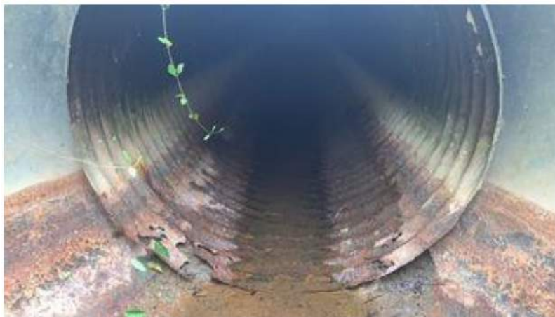
Figure B-1.3-1: Significant Failure Outfall Pipe
