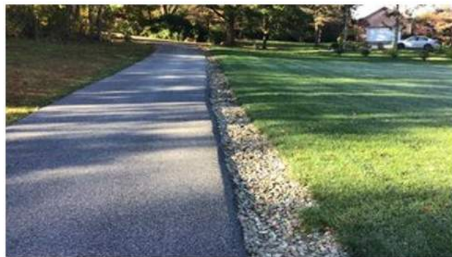
Figure B-3.2-1: Gravel Diaphragm – Transition Strip
