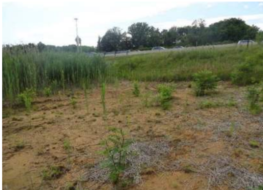
Figure B-4.5-3: Large Area of Bare Soil on Pond Bottom
