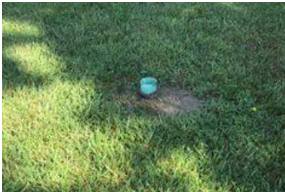
Figure B-6.2-1: Underdrain Cleanout – Cap Missing
