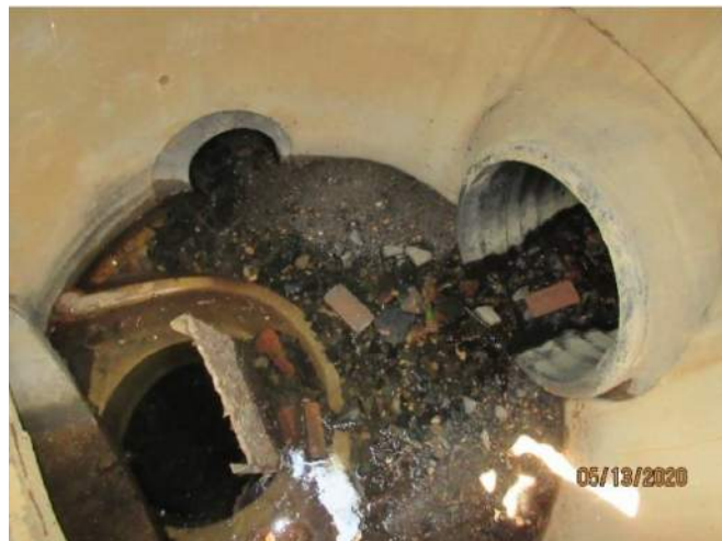
Figure C-2-1: Stormceptor – Accumulated Debris
