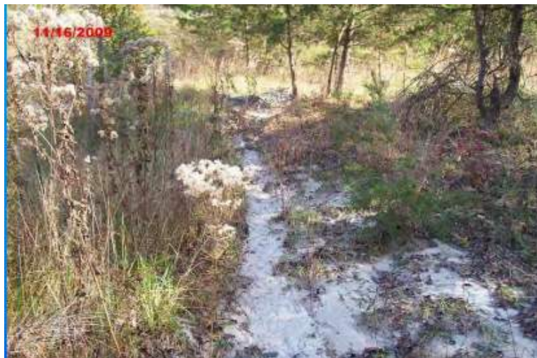
Figure B-5.7-1: Outfall Area Sedimentation
