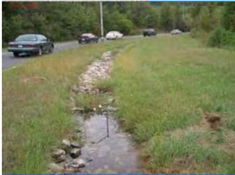
Figure B-4.1-1: Surface Standing Water
