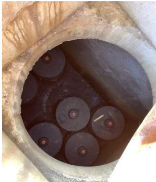
Figure C.1-1: Storm Filter Cartridges
