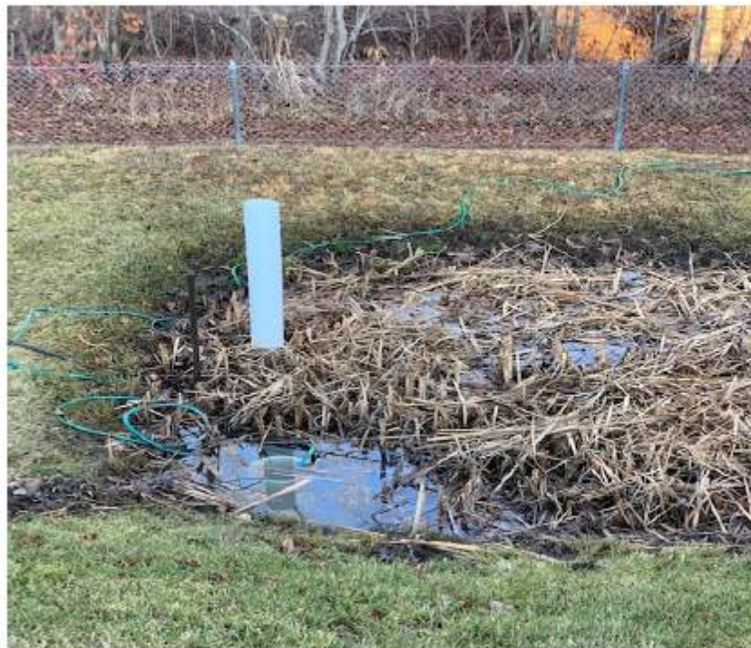
Figure B-3.1.3-1: Forebay Obstructed by Vegetation
