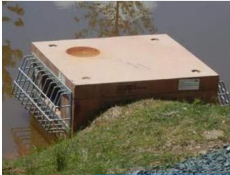
Figure B-5.3-1: Trash Racks on Riser
