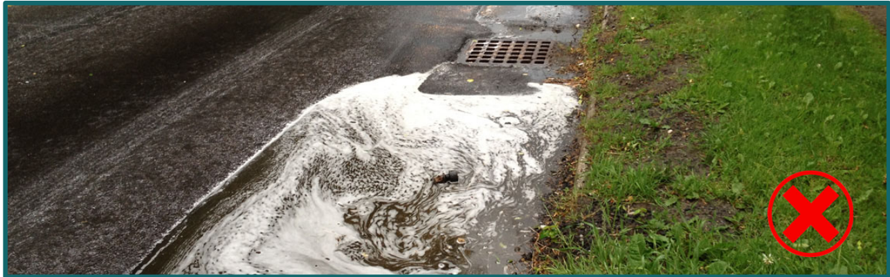
Outdoor Wash Water Discharge to Storm Drain
