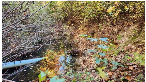
Example of severe erosion and slumping along right bank typical of the end of the restoration. An unknown broken pipe is observed in pieces along the reach.
