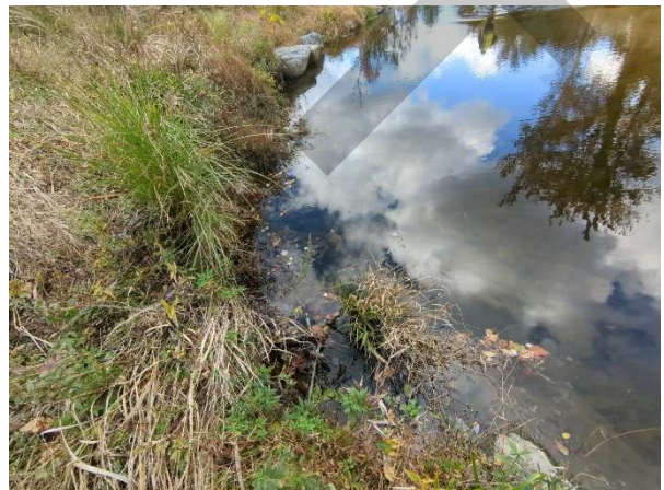
Boulder protection has fallen into stream and bank is eroding at the bend. Near the middle of the restored reach.
