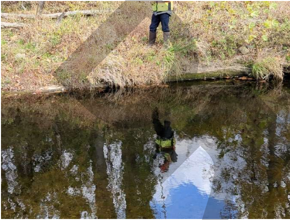
Deep pool under log structure. Currently stable but monitor for possible undercutting.
