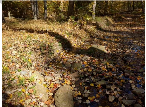
Flanking around riffle structure and subsequent erosion.
