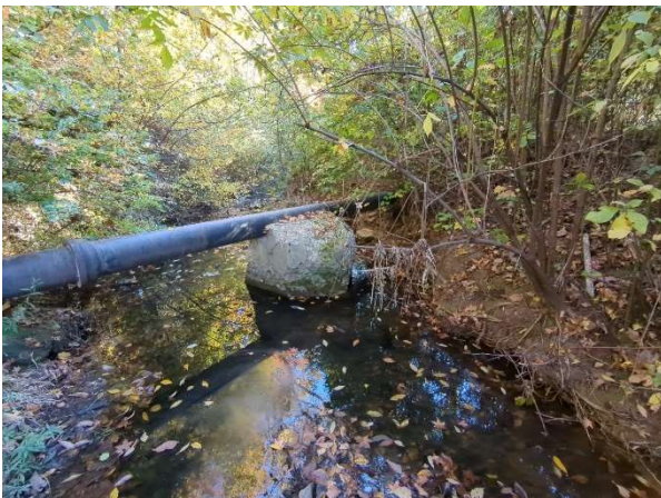
Beginning of erosion and scour near exposed aerial sewer crossing. Mostly on the right bank ~1-3 ft high.
