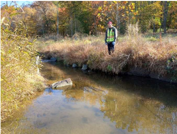
Suspected blown out log structure; causing erosion on left bank
