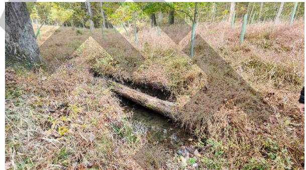
Scour on left bank of log vane. Flow undercutting log; rotting. Stream is stable.
