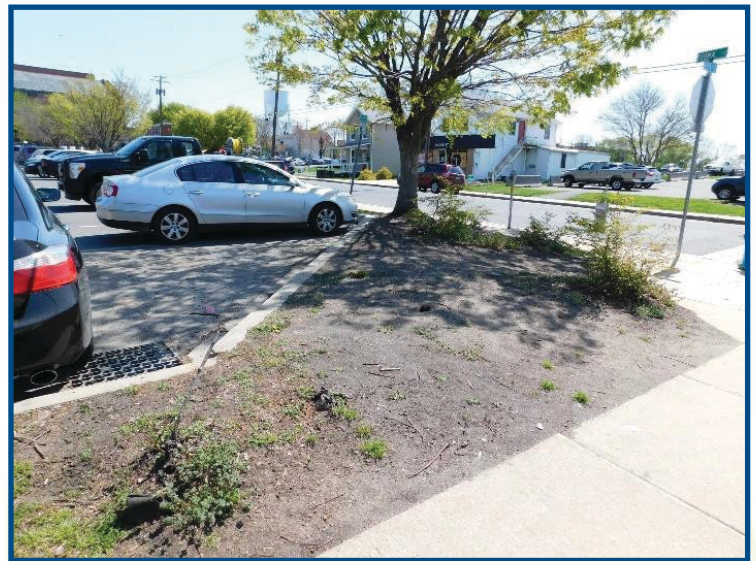
#2 Photo - Corner of parking pavement (with drain) could be retrofitted into contiguous bioretention area with existing planter bed. Trees would be increased longevity with resulting larger soil volume for root growth.
