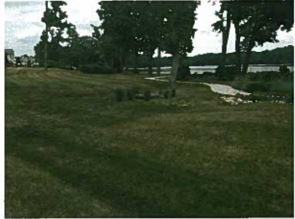
R-SWM0638: Existing sand filter
