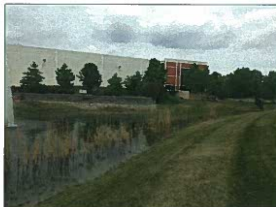
R-NS-4: Pond along Bata Boulevard
