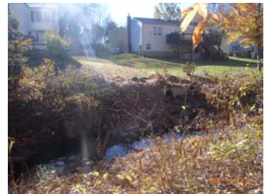
Upstream from Sta 04+25
