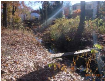
Downstream from Sta 10+25
