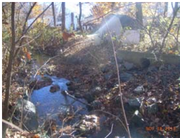
Downstream from Sta 06+00
