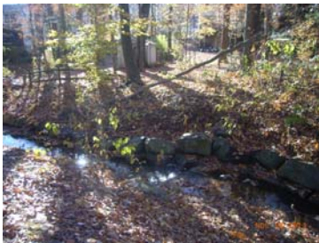
Downstream from Sta 10+75
