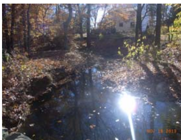
Downstream from Sta 03+20
