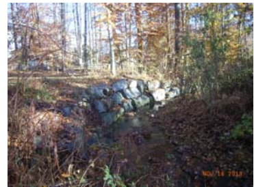
Downstream from Sta 08+75
