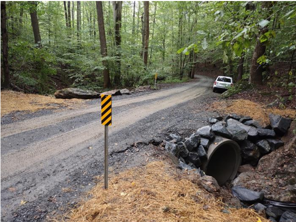
Culvert replaced under Guyton Road in Fallston
