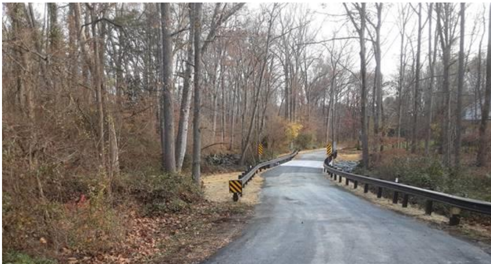
West Chapel Road bridge replacement project completed over Swan Creek
