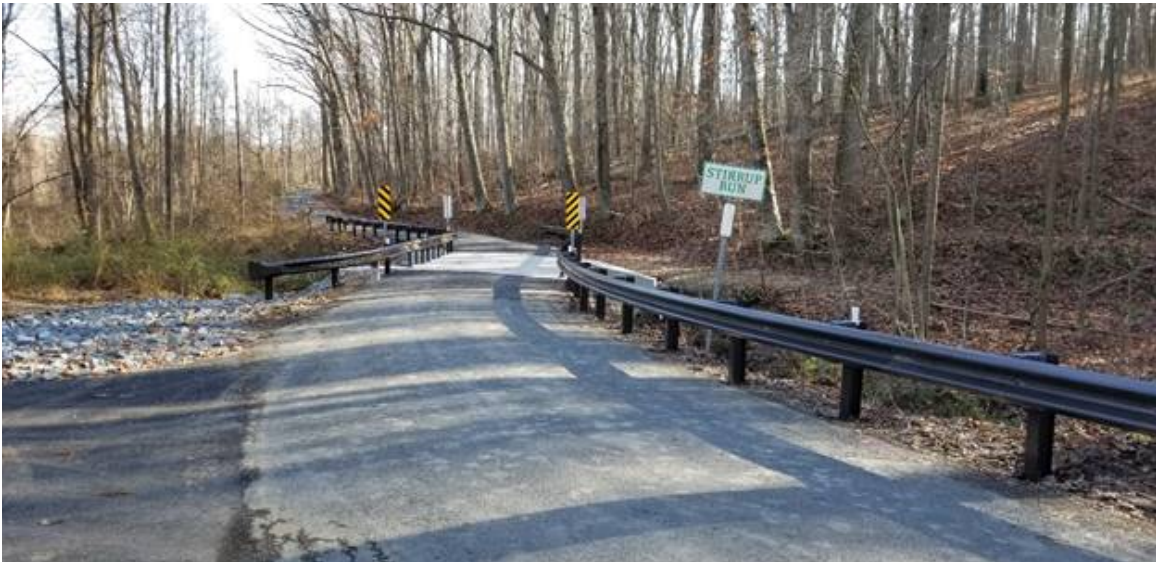
Bailey Road bridge project completed over Stirrup Run
