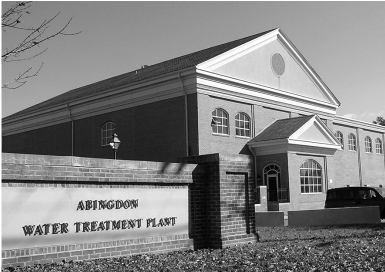
Abingdon Water Treatment Plant
