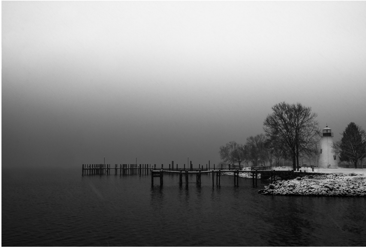
Havre de Grace Pier and Concord Point Lighthouse
