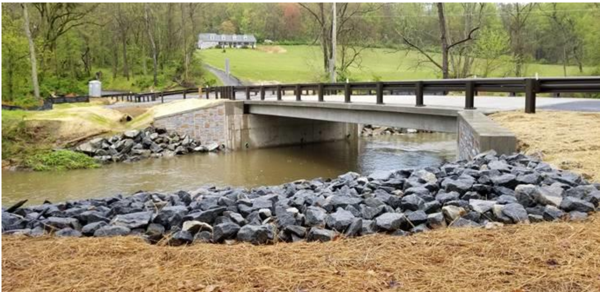
Robinson Mill Road Bridge opened to traffic April 30, 2020
